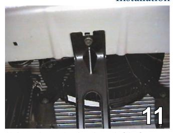
11. Insert the nutplate into the end of the frame to align it with the two back drilled holes. Tighten the 3/8" bolts and lock washers, according to the drawing on page 2.
